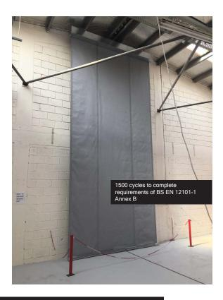
Kent Automatic Smoke Curtains enable the movement of smoke through a building in the event of a fire by channeling smoke to smoke extraction points or creating reservoirs to slow its spread. They remain virtually invisible in their retracted position within the compact headbox in its retracted position within the compact head box. When signalled by a local detector or alarm, they descend to the operational level above the floor.
